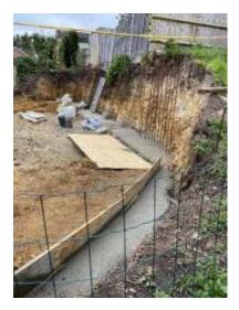
**1.1.2** The rebar spacing is not according to the plan, only 2/3 the required number of upstand elements have been used.
