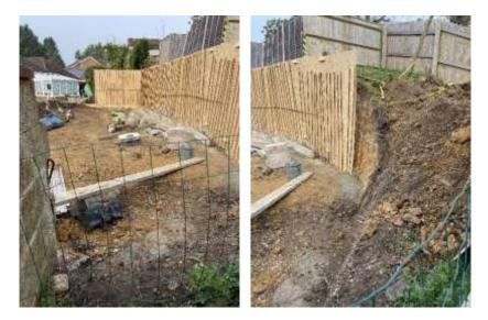
They can be counted in these photos which were sent to council. Moreover, the upstand rebar was specified as 16mm. No evidence that 16mm rebar has been used is available and discarded scrap is 12mm (half the cross sectional area / half the reinforcing strength) so potentially  $2/3 \times 1/2 =$  only 1/3 of required level of reinforcement. Development is demonstrably not according to the submitted plan but the Officer claims it is. Why?
